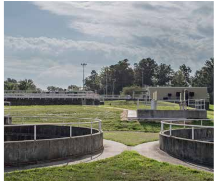
MSD's Hite Creek Water Quality Treatment Center will expand to accommodate growth in northeastern Jefferson County. MSD will spend $8 million on this effort in the next 12 months.
