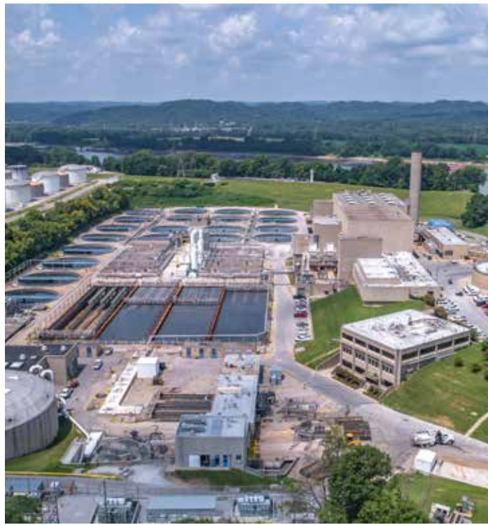
MSD's Morris Forman Water Quality Treatment Center is Kentucky's oldest and largest—by volume—wastewater treatment center in Kentucky. It went into service in 1958 and some of those 60 year old parts are still in service. The facility is slated to receive $5.7 million in improvements in the next 12 months.
