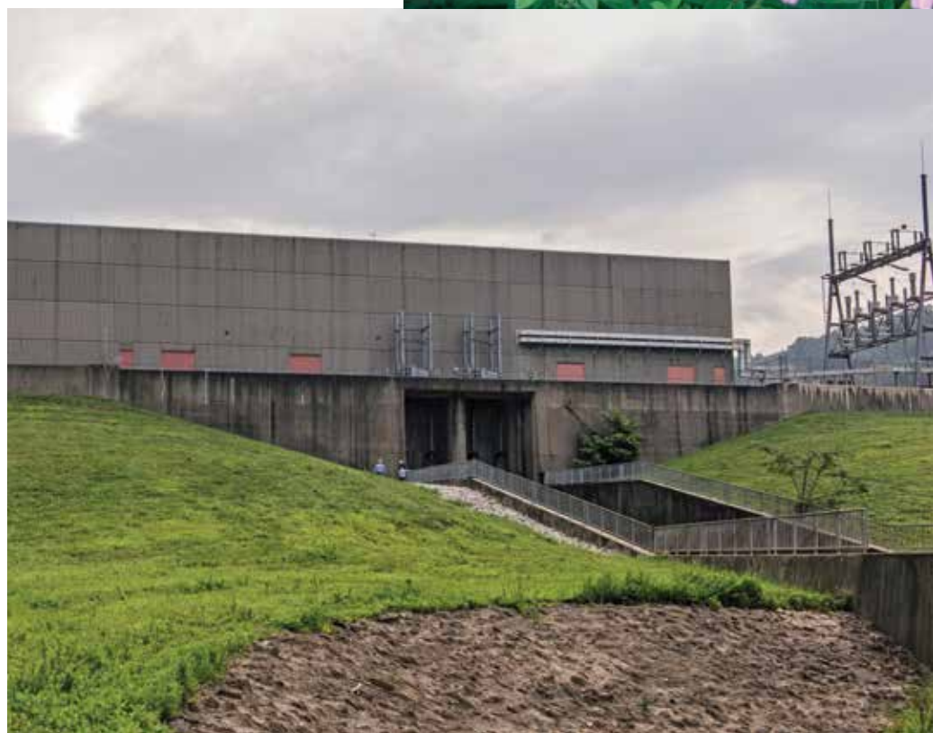
Above: The Pond Creek Flood Pump Station, part of the Southwest Extension of the Flood Protection System, can move more than 1.8 million gallons of water per minute.
