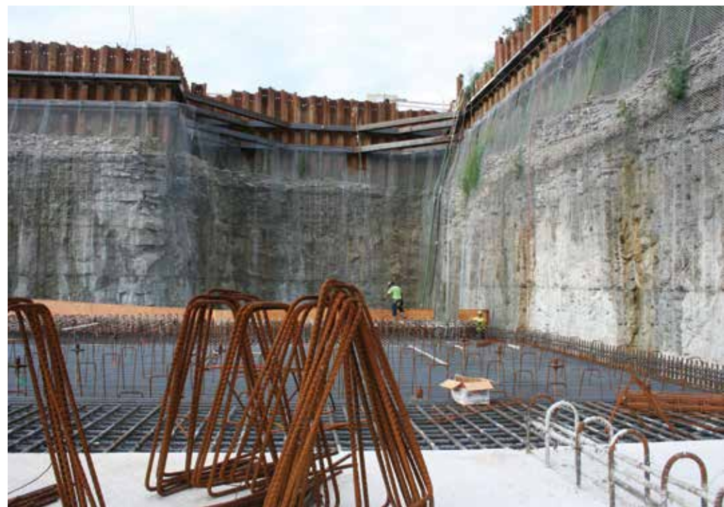
Above: Construction is underway for the Logan Street Basin and is scheduled for completion in late 2017. This basin will offer Beargrass Creek and area residents protection from combined sewer overflows.
