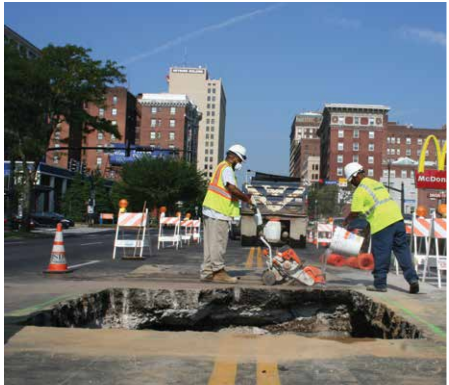
Above: MSD Crews work to repair a Broadway Trunk Sewer collapse.
