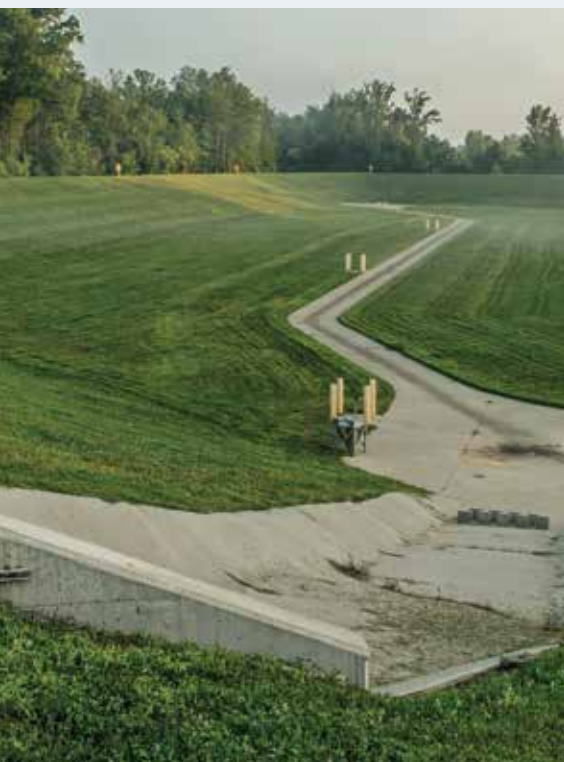
Above: Stormwater basins, such as this one in far southwestern Jefferson County, reduce wet-weather sewer overflows and decrease pollution in local waterways by providing storage during wet weather.
