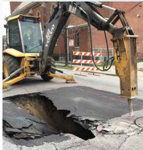
Crews work to repair a sewer collapse at Clay Street and Muhammad Ali Boulevard.
