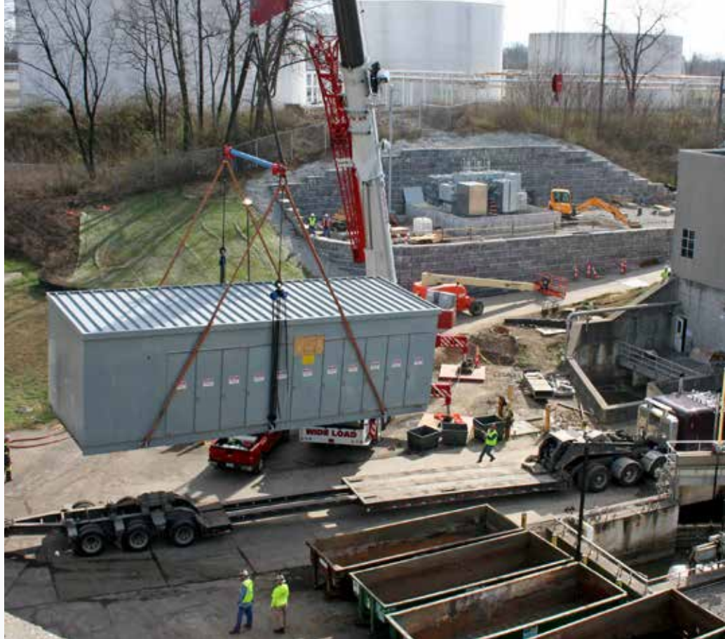
The new high-yard switch house is lifted from the transport truck bed.
