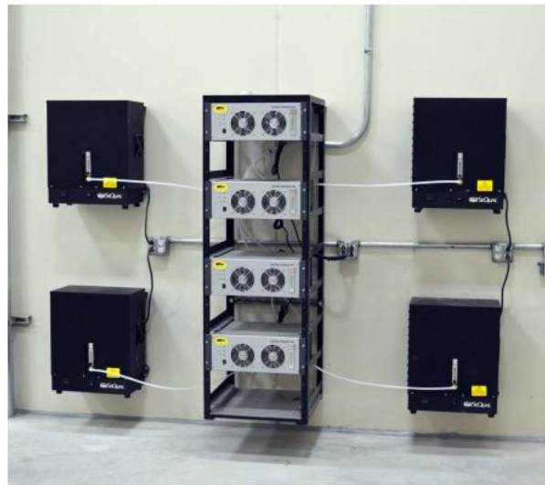
Ozone Generators/Oxygen Concentrators (typical configuration)
