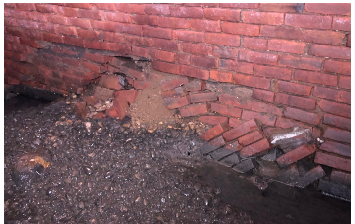
Fallen bricks and debris block the flow inside the sewer line under E Broadway.
