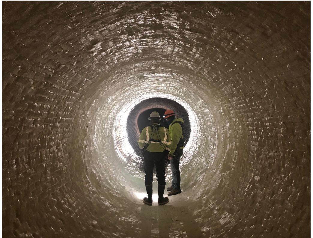
Workers stand inside a recently repaired section of the brick sewer pipe under East Broadway, which dates to 1866. An epoxy spray coating will add years to this sewer line's useful life.
