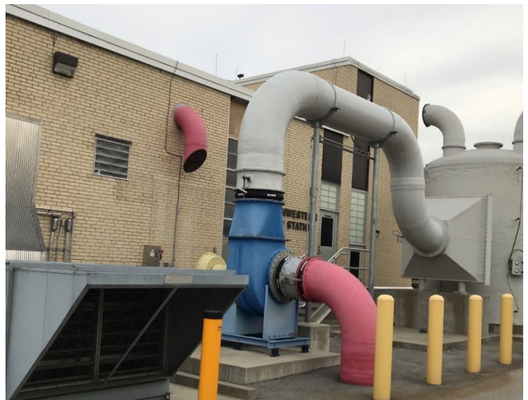
Figure 3-16 Pump Station 5 Odor Control System
