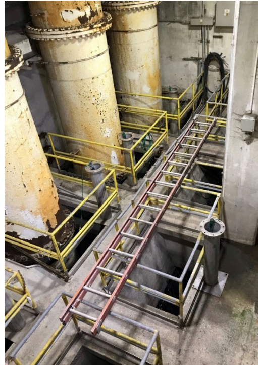
Figure 3-11 Pump Station 4 Wet Well Intake
