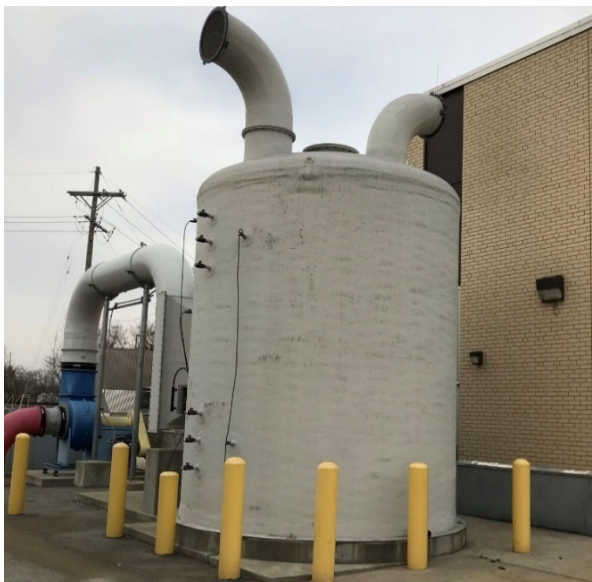
Figure 3-16 Pump Station 5 Odor Control System
