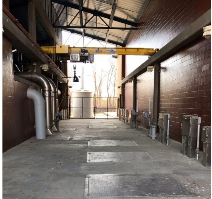
Figure 3-7 Pump Station 3 Wet Wells (L) and Valve Vault (R)
