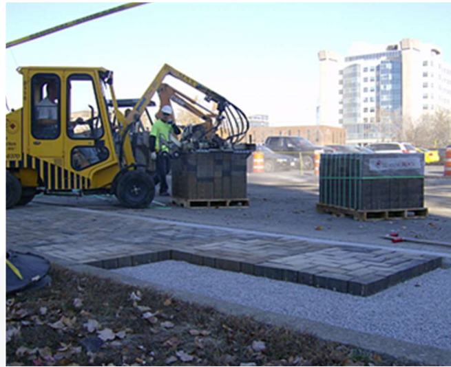
Mechanical installation of permeable interlocking concrete pavers
