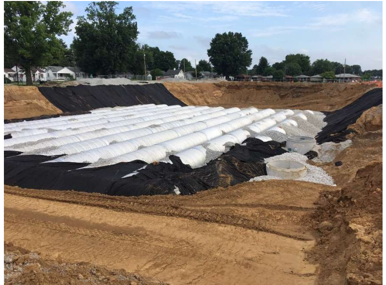
Underground Infiltration Basin at Churchill Downs
