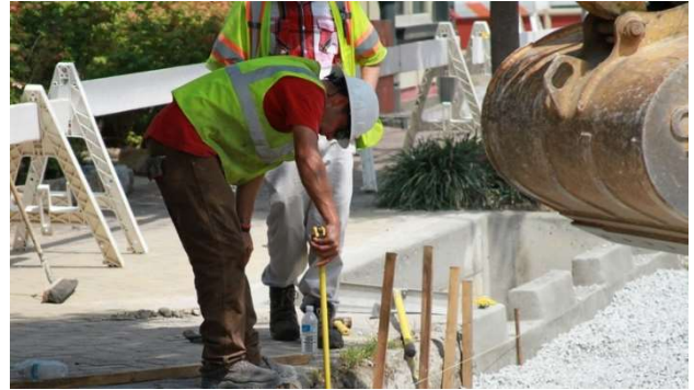
Construction of permeable paver parking lane and tree boxes
